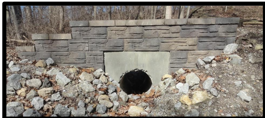
New erosion control riprap
